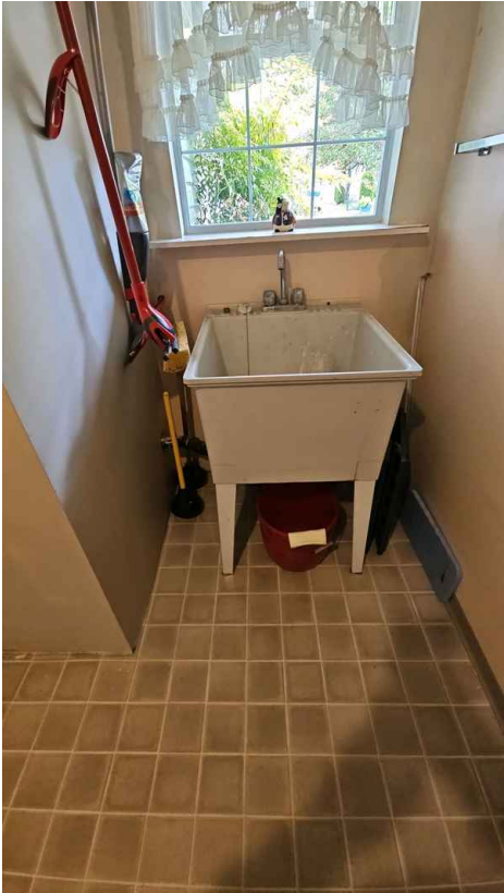
Laundry unit: Laundry Sink
