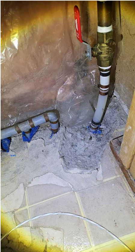
Main Water Service: Main supply line material Pex, Poly-B
