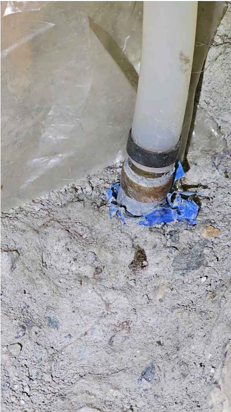
Main Water Service: Main supply line material Pex, Poly-B
