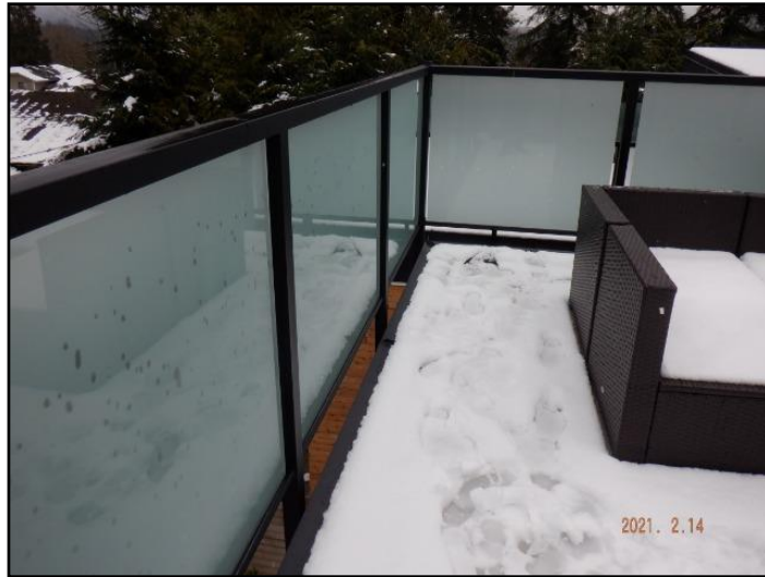
8. Metal and Glass Railing
