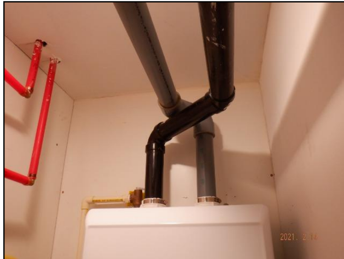
27. Direct vent - sealed combustion
